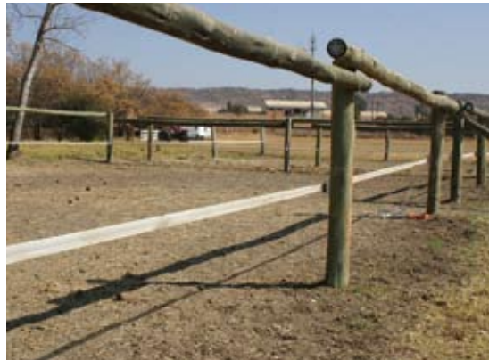
A well-constructed wooden fence. It would, however, have been better to have the rails on the inside of the posts. This would minimise the chances of injury even more
